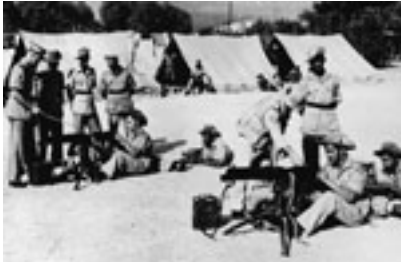
Reinforcement of the Cape Documentation Centre, Pretoria)
